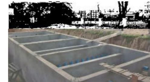
**DEWATS SYSTEM** under the toilet block to convert grey/black water to fresh water which again can be used for flushing and irrigation
