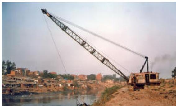
6.5 km of the NG Drain has also been deepened, impounding 155 MG water annually and a further 2.3 km is proposed to be deepened by 1.5 m. The Mungeshpur drain has been regraded in 12.5 km impounding 4 MG water:
