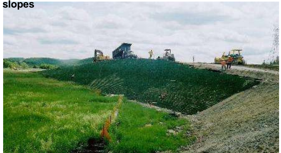
Planting the slopes with grasses and other plant material prevents erosion on shallow slopes.
