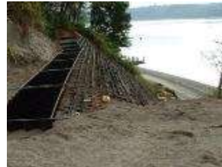
Geo – grid method for soil stabilization of the existing nallah slopes
