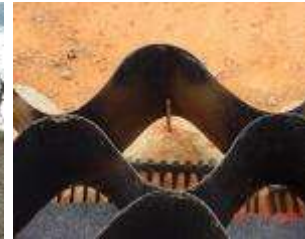
Geo – grid method for soil stabilization of the existing nallah slopes
