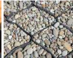
Geo – grid method for soil stabilization of the existing nallah slopes
