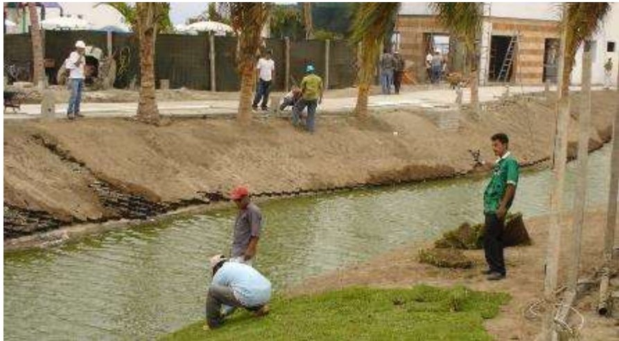
Planting the slopes with grasses and other plant material prevents erosion on shallow slopes.
