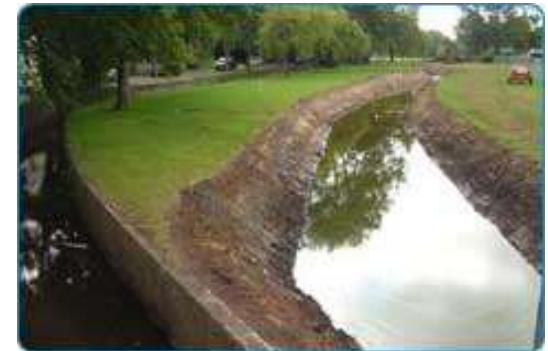
Planting the slopes with grasses and other plant material prevents erosion on shallow slopes.
